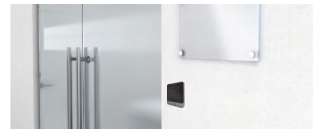
FRONT DOOR (EMPLOYEE)
